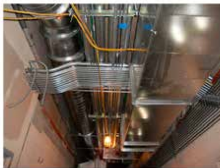
Basement corridor installed
